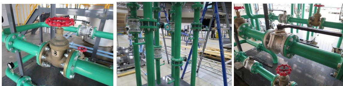
左から：Ball Valve, Rubber Seated Valve, Gate Valve
